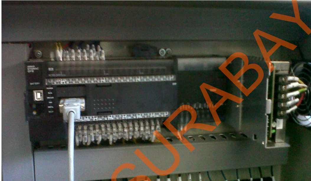
Gambar 4.9 PLC Omron ( mengontrol mesin outomatic mixing di pabrik pipa PVC).
