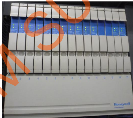
Gambar 3.15 Process Manager I/O
