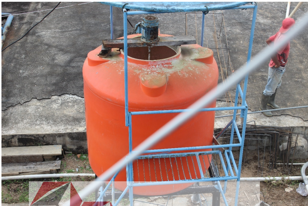
Gambar 4.7 Dokumentasi Bak Pencampuran Soda as dan Clorofit
