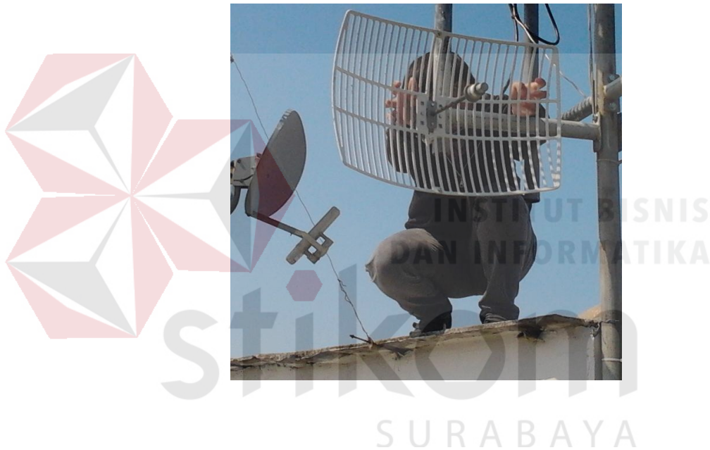
Gambar 4.5 antenna grid ( frekwensi 5,8 GHz 27 db)
