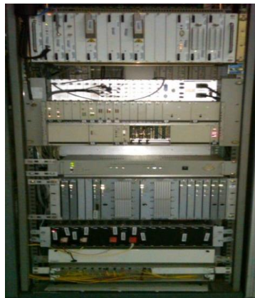
Gambar 3.7 Modul Radio NEC DMR 3000S (SDH)
