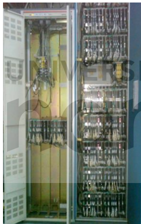
Gambar 3.6 Modul Multiplex PDH
