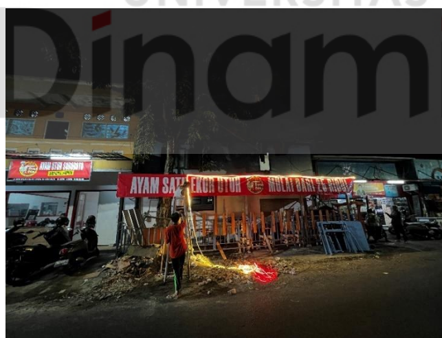
Gambar 4.12 Pemasangan Lampu LED
