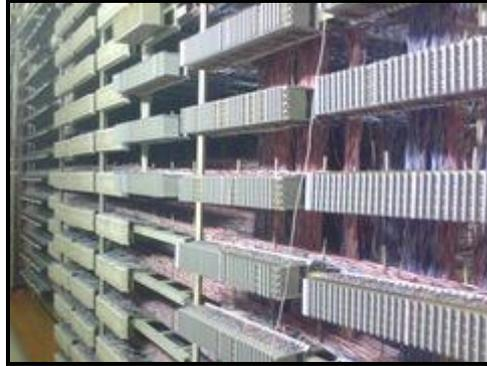
Gambar 3.7 Terminal Blok Horizontal
